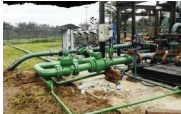
Tie-in Point to Trans Niger Pipeline
