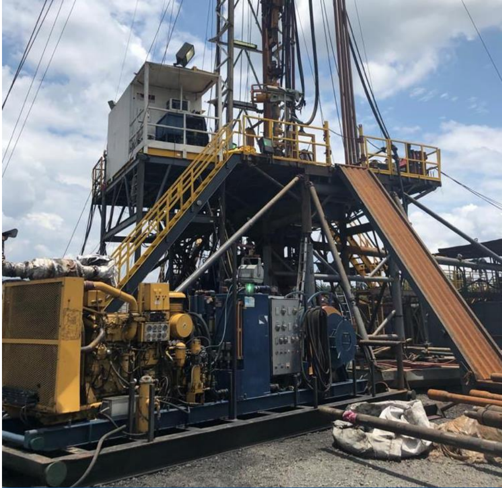
Oza-1 drilling rig finishing re-entry
