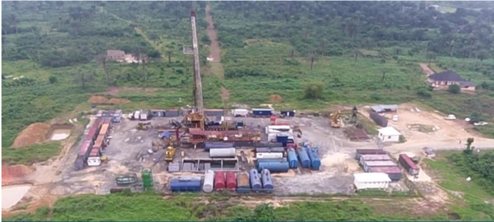
Oza-1 drilling rig and pad
