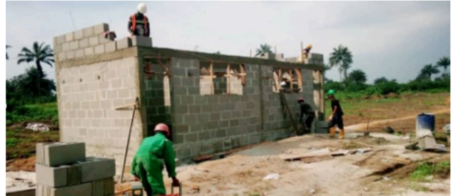
Construction of on-site staff housing
