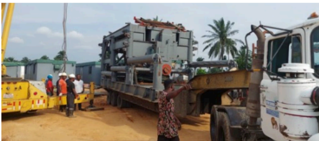
Oza-1 drilling rig arriving on site
