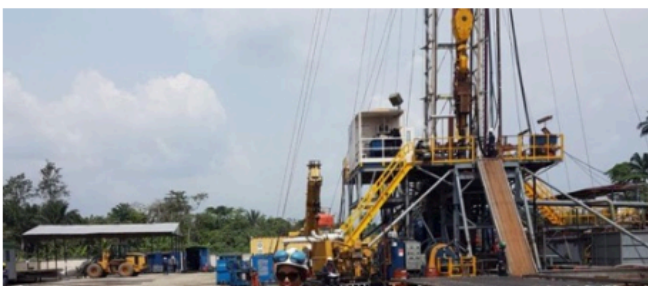
Oza-1 drilling rig assembled and ready on drilling pad
