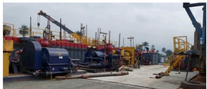
Oza-1 drilling rig equipment assembled and ready
