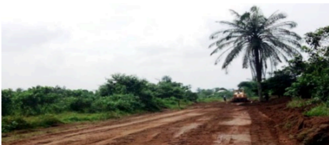
Access road cleared for rig mobilization
