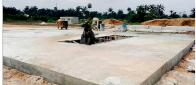
Completed foundation for Oza-1 drilling pad
